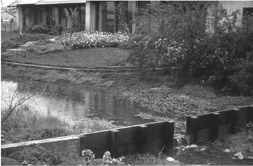
Figure 8.19 Natural or “open” drainage systems, such as that shown here, in the author’s neighborhood of Village Homes, return many ecological functions to the residential landscape. Photograph by Robert Thayer.
