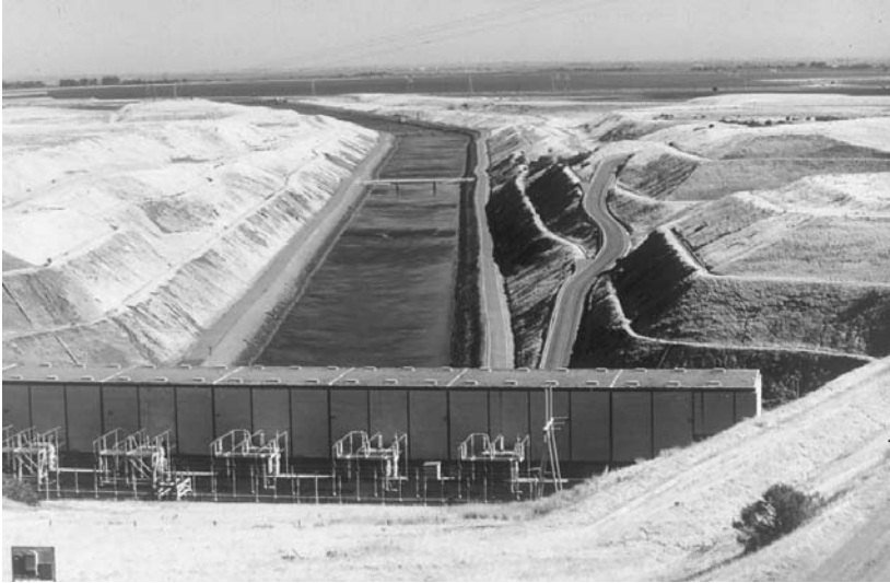
Figure 7.2 The State Water Project's Harvey O. Banks Pumping Station, near the Sacramento–San Joaquin Delta, is an example of large-scale, one-dimensional infrastructural planning. While its foremost purpose is delivery of irrigation water southward, it also contributes to altered channel flow directions, increased salinity, and loss of anadromous fish populations in the delta, as well as considerable energy consumption. Photograph by Robert Thayer.
