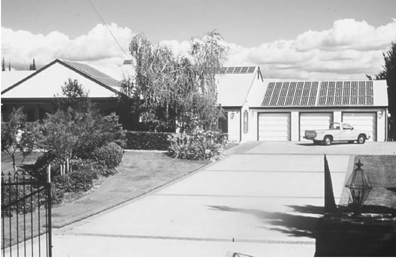
Figure 8.18 The best untapped source of clean, renewable energy for the Sacramento Valley is the rooftops of its buildings. Photovoltaic electric panels provide a majority of the electrical energy needed by this residential dwelling. Photograph courtesy of the Sacramento Municipal Utility District.
